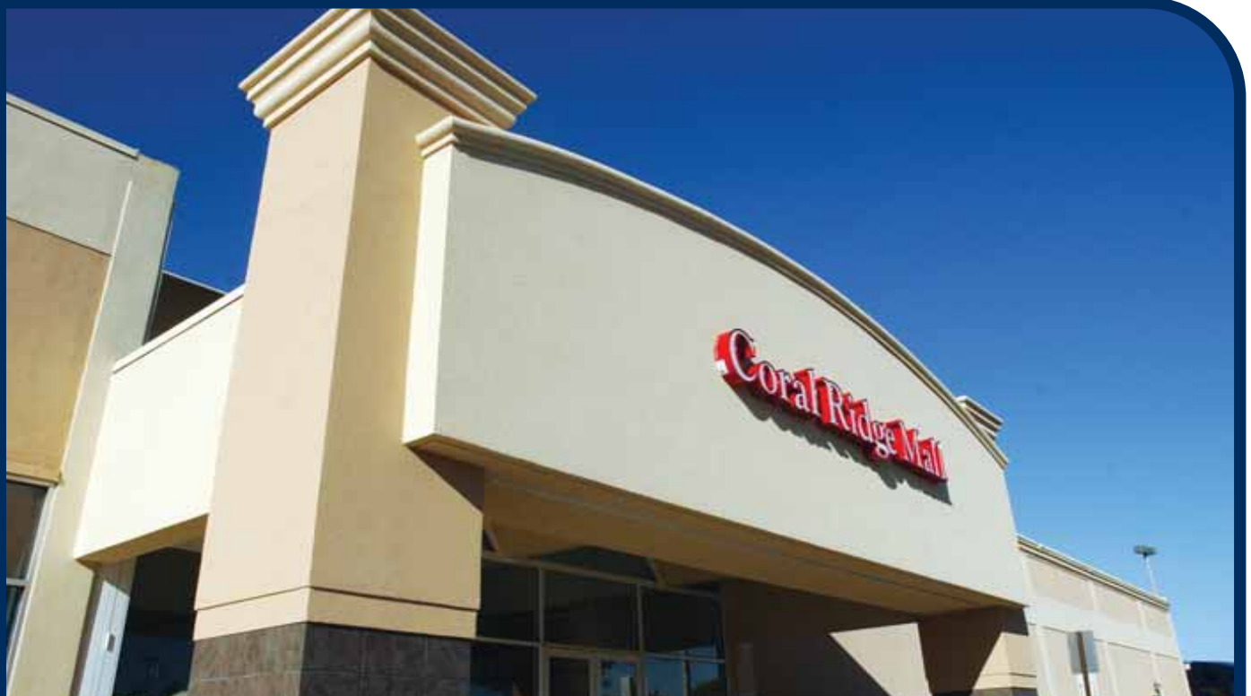
Project Featured: Renovated Northeast Entrance at the Coral Ridge Mall Shopping Center in Fort Lauderdale
